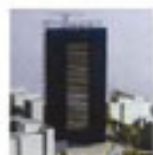
26-storey apartment building near Columbus shopping centre
